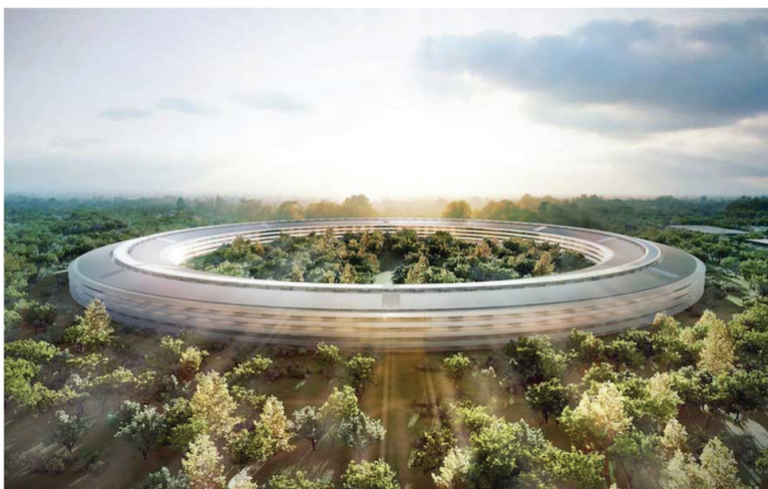
2. Apple Park, Cupertino, California, 260,128 square meters. Apple's new corporate headquarters is a four-story, ring-shaped building, with a circumference of 1,512 sq ft. It houses 12,000 employees and opened in April 2017. It was designed by Foster and Partners. In addition to the four floors above ground, it also includes three stories below ground. The building sits on top of 700 base isolators. Each isolator is 7 ft in diameter and weighs about 15,000 lbs. The isolators were customized for low friction, according to the lead structural engineer, John Worley. Construction of the entire Apple Campus 2, including the headquarters building as well as a 1,000-seat auditorium (the Steve Jobs Theater), a wellness-fitness center, two R&D buildings, a visitor center and parking structures, totaled $5 billion. The building's inner part is a 30-acre park, featuring fruit trees, winding paths and a pond.
